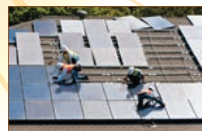
4) Solar panels are positioned and connected to the wiring harness.
