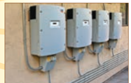
5) Inverters convert direct current (DC) from the panels into alternating current (AC) and pass back to the Smart Meter from PG&E.
