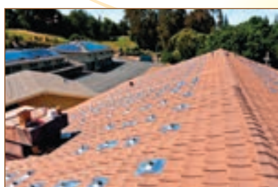
1) Mounting bolts and watertight flashing are attached to roof structure
